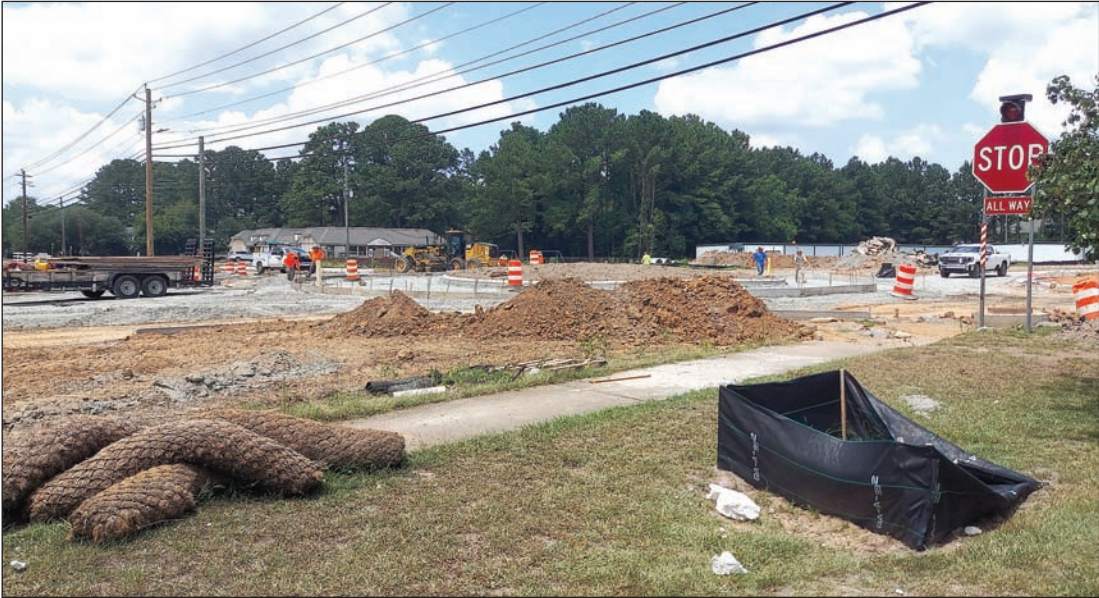
Construction workers are on pace to have the roundabout at the Claxton Dairy Road/Woodlawn Drive intersection opened for traffic by the end of this month/PAYTON TOWNS III
