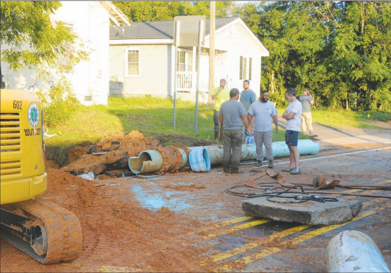
Dublin City Manager Josh Powell (right) talks to a city work crew repairing the broken water main on Joiner Street/KYLE DOMINY
