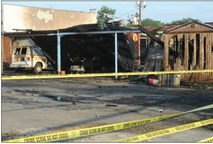
The fire gutted the Proline Commercial Services building while also destroying equipment and several vehicles /PAYTON TOWNS III
