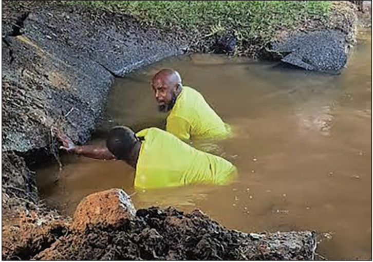
City workers dive in to repair the water main break on Joiner Street/SPECIAL PHOTO, City of Dublin
