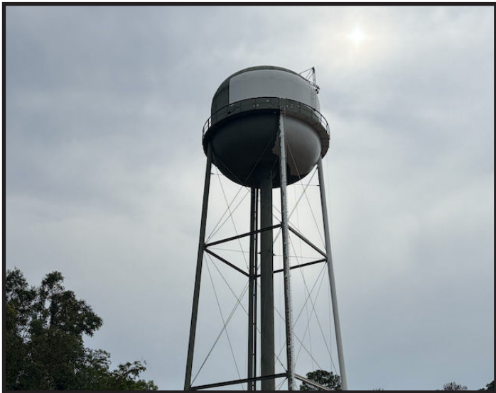
The water tower on Old Gordon Road is currently in the process of being painted/CAROLINE WEATHERSBY
