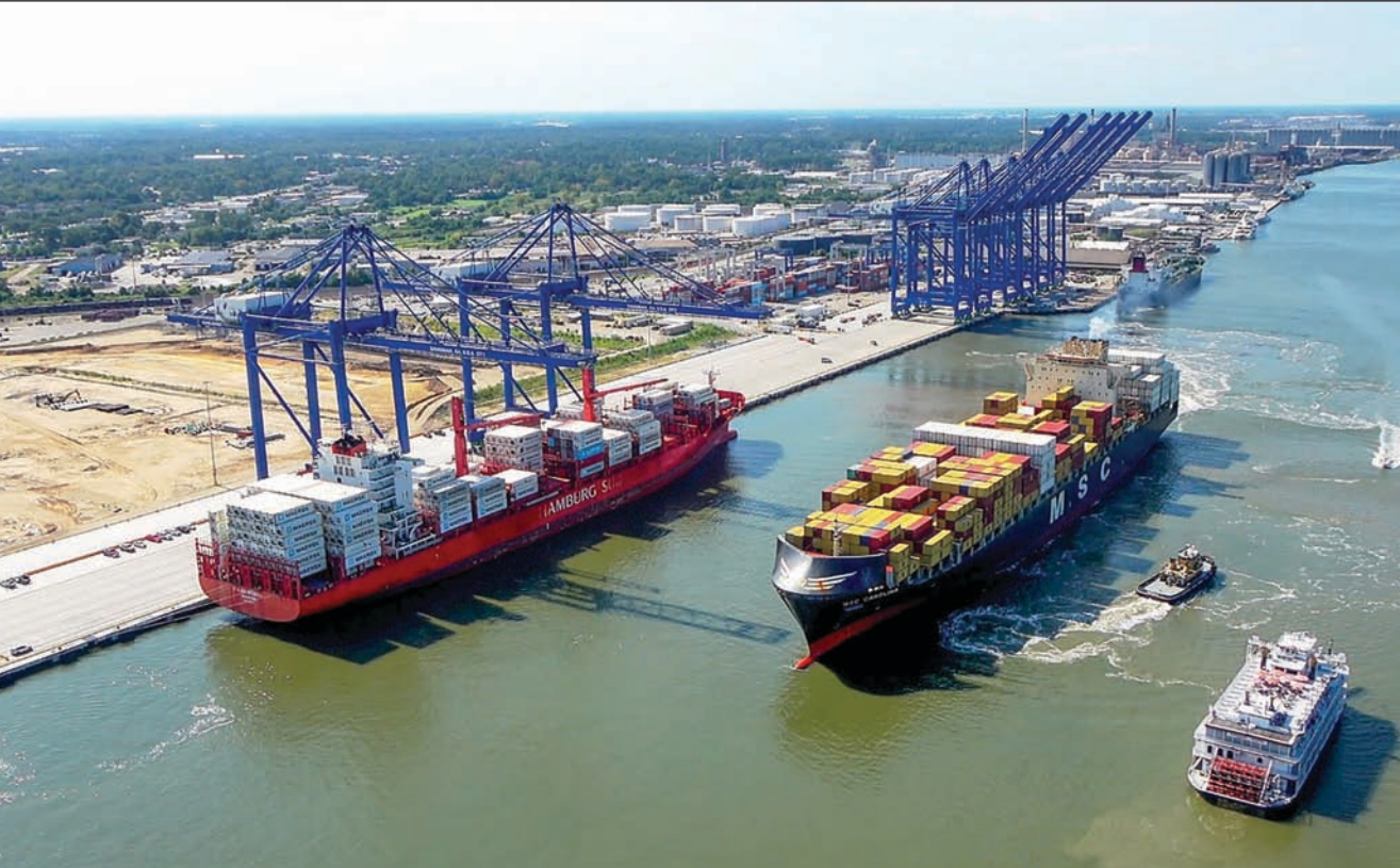
The Port of Savannah's Ocean Terminal now has a 2,650-foot berth ready for two large ships/SPECIAL PHOTO, Georgia Ports Authority
