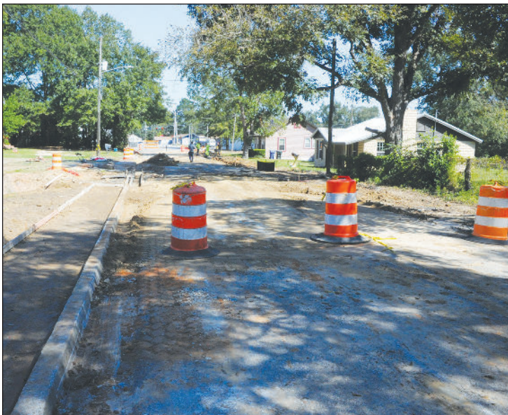
Sidewalk was closed and being constructed/PAYTON TOWNS III
